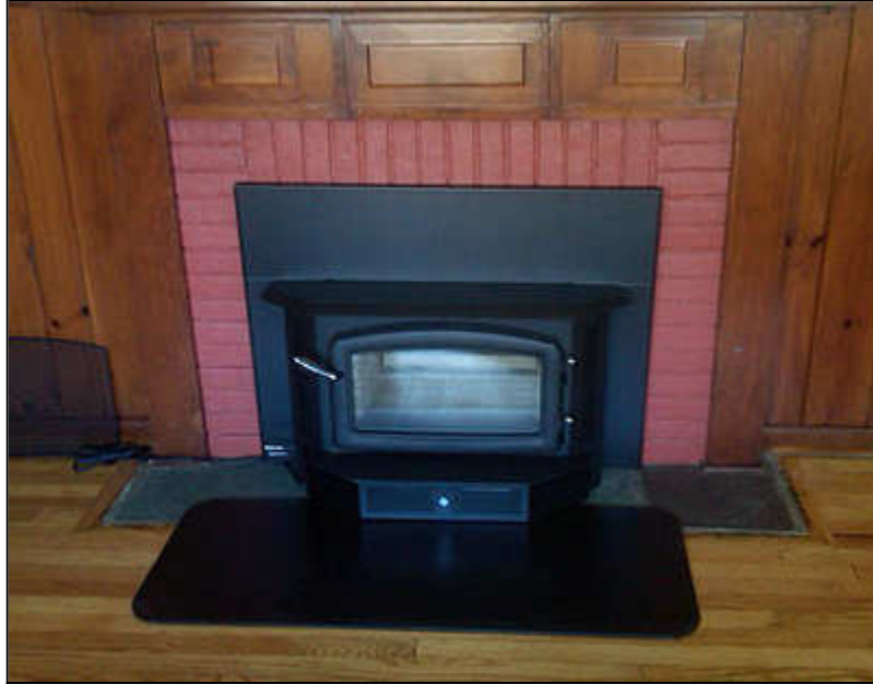
Regency I2400 installed with hearth pad
